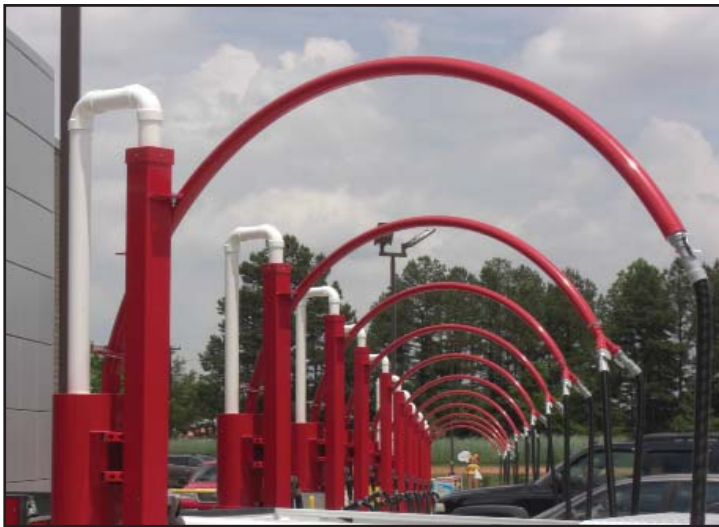
9' Vacuum arches with inground PVC piping.
