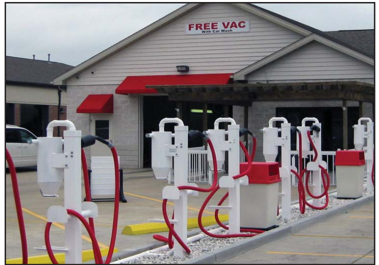
Vacuum stanchions with in-ground piping system.
