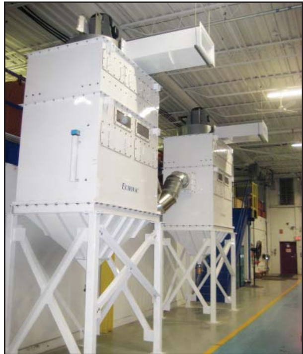
Type "B" Central Wet Collectors - Drain Valve Dust Removal
