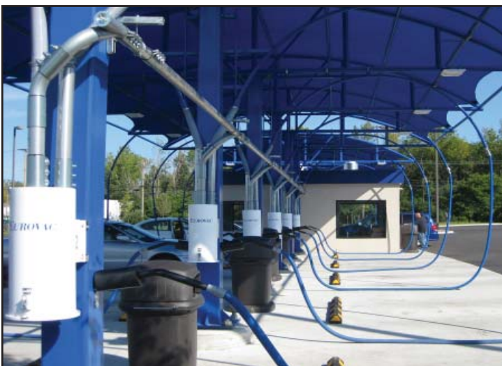
Arches under canopy structure with aluminum tubing and compression couplings
