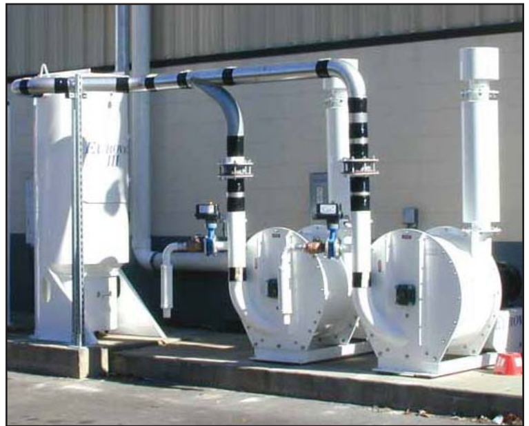
Eurovac III Double Pump System 10HP - 75HP (x 2) Centrifugal Multi-Stage Pumps and Bag Filter Separators
