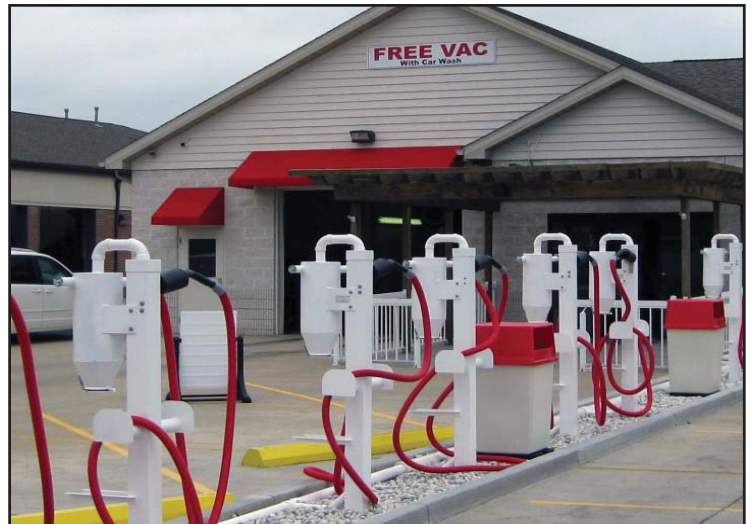
Vacuum stanchions with in-ground piping system
