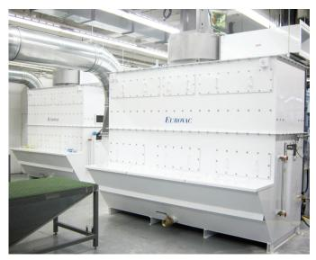
Type "A" Central Wet Collectors - Sludge Rake Dust Removal
