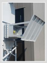
Explosion vent with deflector to divert blast upward thus minimizing possibilities of personal injury or property damage
