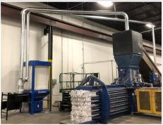
Manual shaker open type collector with side floor mount radial blade fan and low profile canister (interior installation only)
