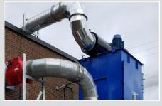
Fan outlet silencer to recycle clean air back in to the facility. Isolation valve (red) to prevent fireball from coming back thru the main ductwork
