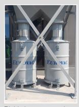
Rigid clamp connection from hopper to drum lid. Drum dollies on casters for easy movement of drums when full
