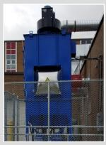
Stainless steel rupture disk with weather cover for ST2 type dusts
