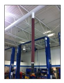
Telescopic drop systems have three difference size hoses interconnected to work as one. The smaller hoses are housed inside the larger hose and are held in place by a manual support bracket when system is not in use. To use, simply raise the bracket to release and drop the hose.
