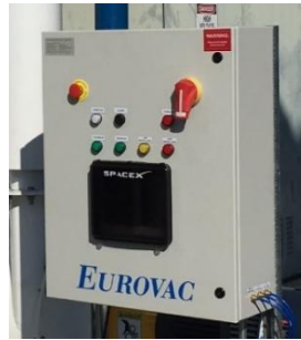
PLC Control Panel
